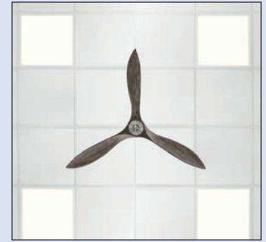
Fig. 9: Especially at workplaces, the flickering of ceiling fan blades running through the lighting is disturbing. This should be taken into account during planning.
